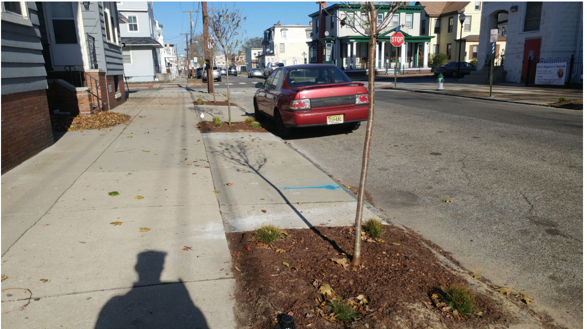
Planted stormwater tree beds designed to capture runoff from the sidewalks; photographed by planting volunteer in the fall of 2019.
