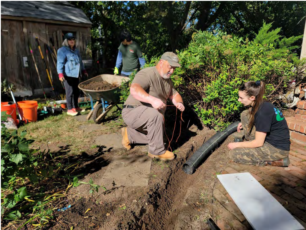
Installation included connecting a downspout to direct stormwater into the rain garden
